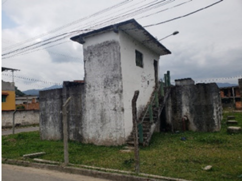
FIGURA 6-12 – ETE FRANCISCO GUEDES – VISTA GERAL
